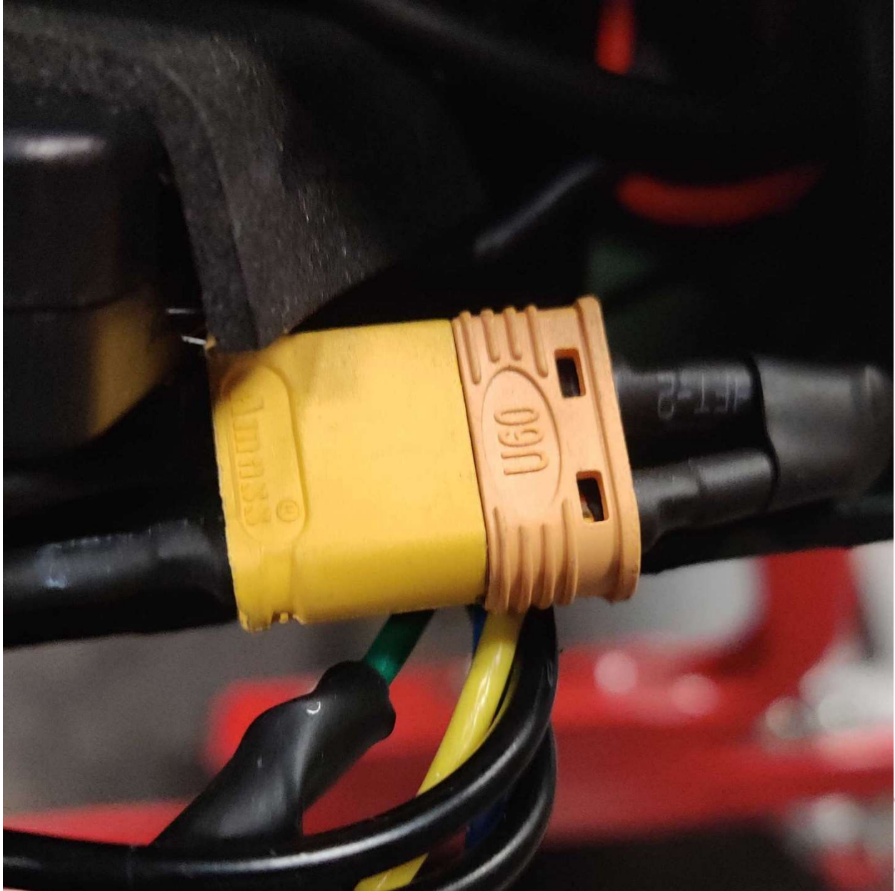
Figure 2b: Battery wire
