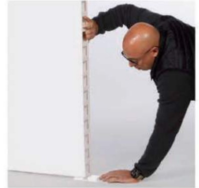
Placing an Inter-Panel Connector (2 Way) underneath an EverPanel
