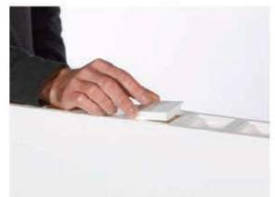
Installing Finishing Caps on an EverPanel
