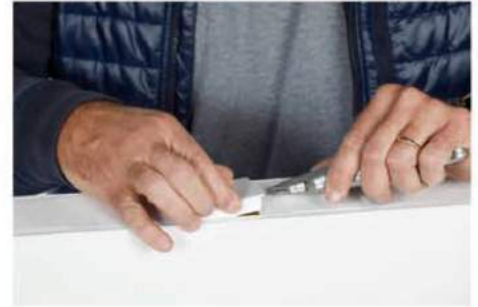
Removing a Finishing Cap using a knife blade
