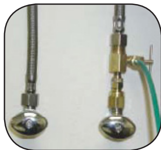
INSTALL ON COLD WATER LINE
